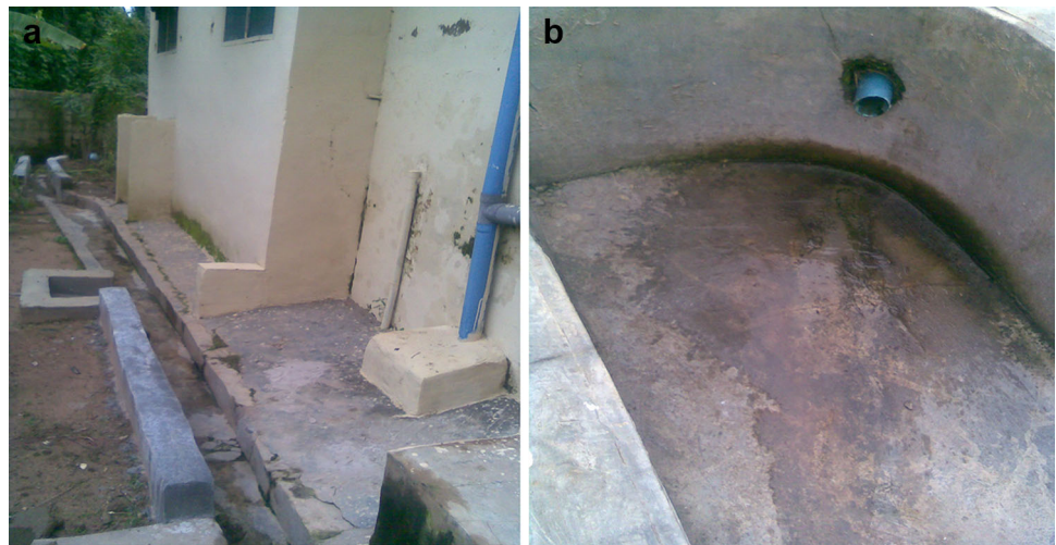
Fig. 2 a Discharge of wastewater from bathroom in a Peri-Urban System. b Discharge of wastewater from the kitchenette
